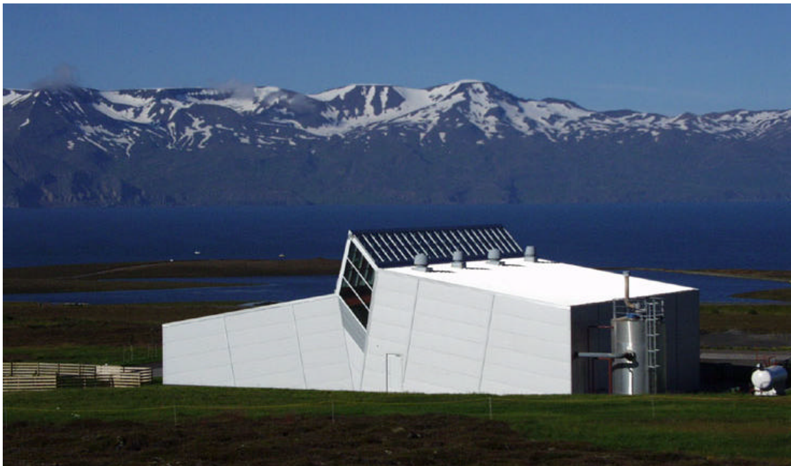
Picture 4. The new “Kalina” low-heat power plant in Husavik.
